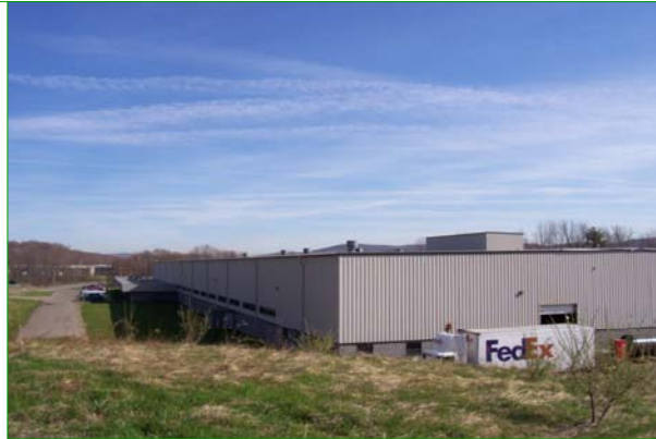
Samscreen Incorporated's Manufacturing Facility Located in Conklin, New York.
